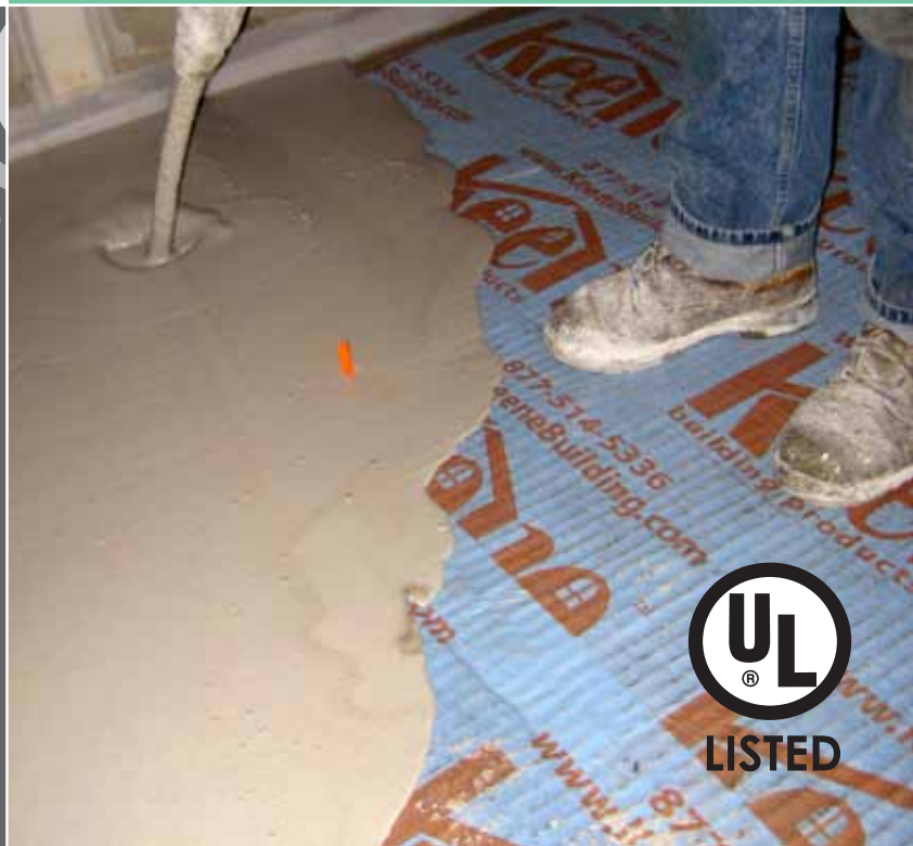
Photo: Gypsum concrete being poured on Quiet Qurl®
